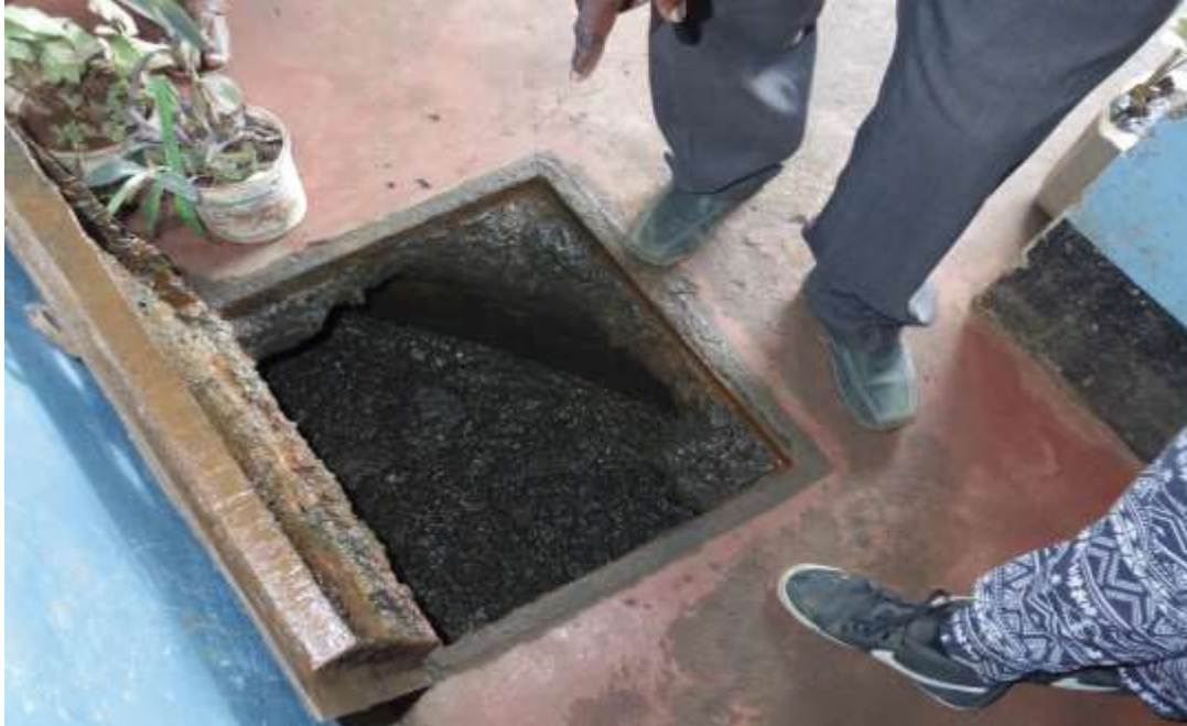
Sewer at the KIDYOT
