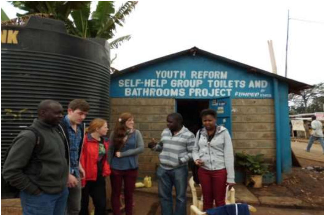
Impressive Sanitation Project in Kibera
