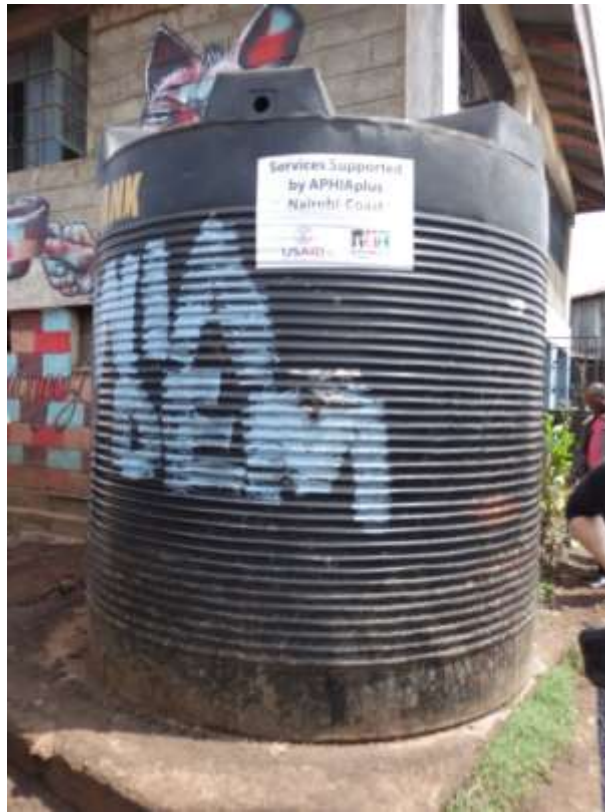
Water tank provided by the Nairobi Water Company
