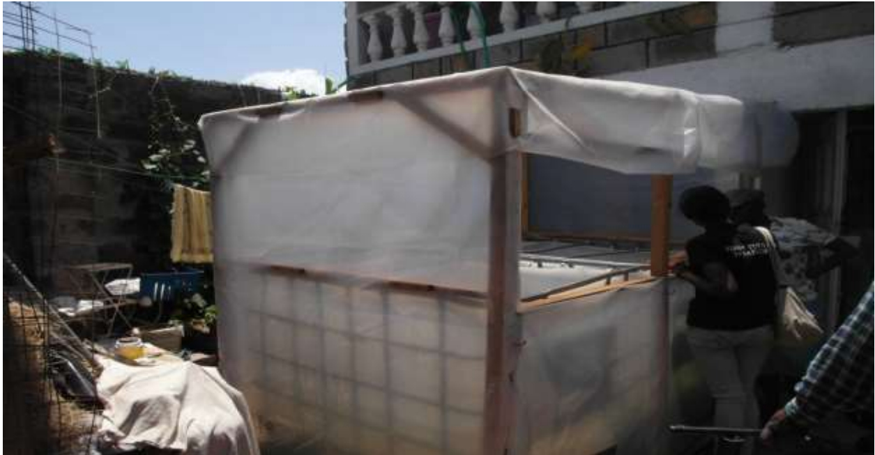
Aqua farming construction, at Sara Itambo's farm in Donholm
