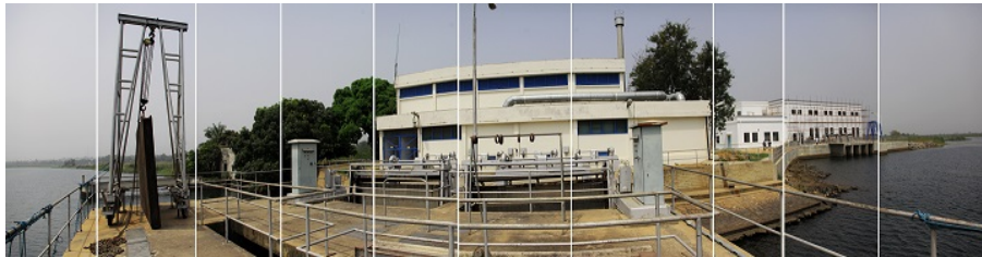
Figure 9 – Kpong Treatment Plant © WaterPower, 2015.
