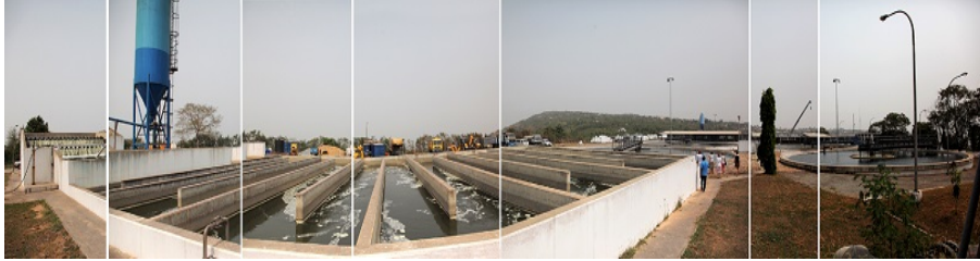
Figure 8 – Weija Treatment Plant © WaterPower, 2015.
