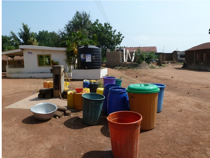
Figure 11- Standpipe and polytank in Abokobi © WaterPower, 2015.
